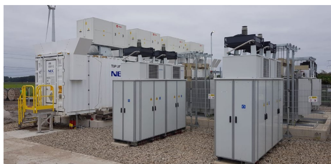
Figuur 4.1 GIGA Rhino battery container on site
